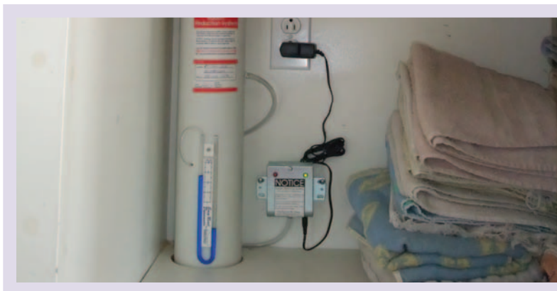
Photo 11 - Two devices used to insure the functionality of the soil depressurization system: a pitot tube and an audible alarm
