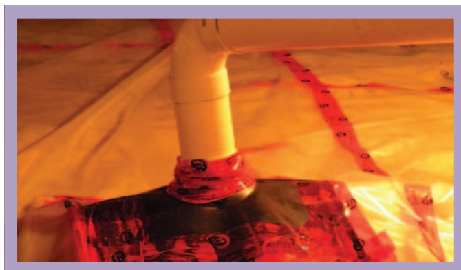
Photo 5 – Sealing the penetration through the membrane
